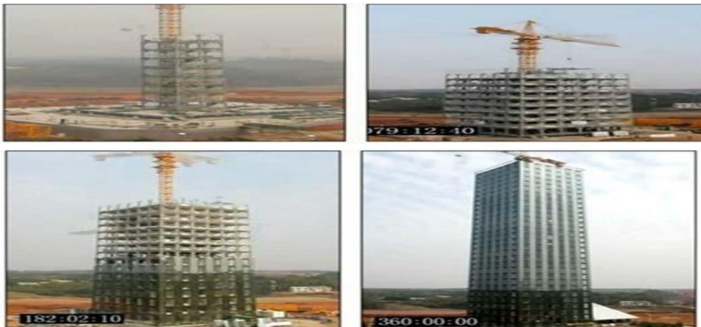
Fig.12 Overview of the rapid constructed 30 storey hotel building construction process (Sources; A Chinese Miracle 30-storey hotel in 15 days... http://thefabweb.com/16814/a-chinese-miracle-30-storey-hotel-in-15-days )
